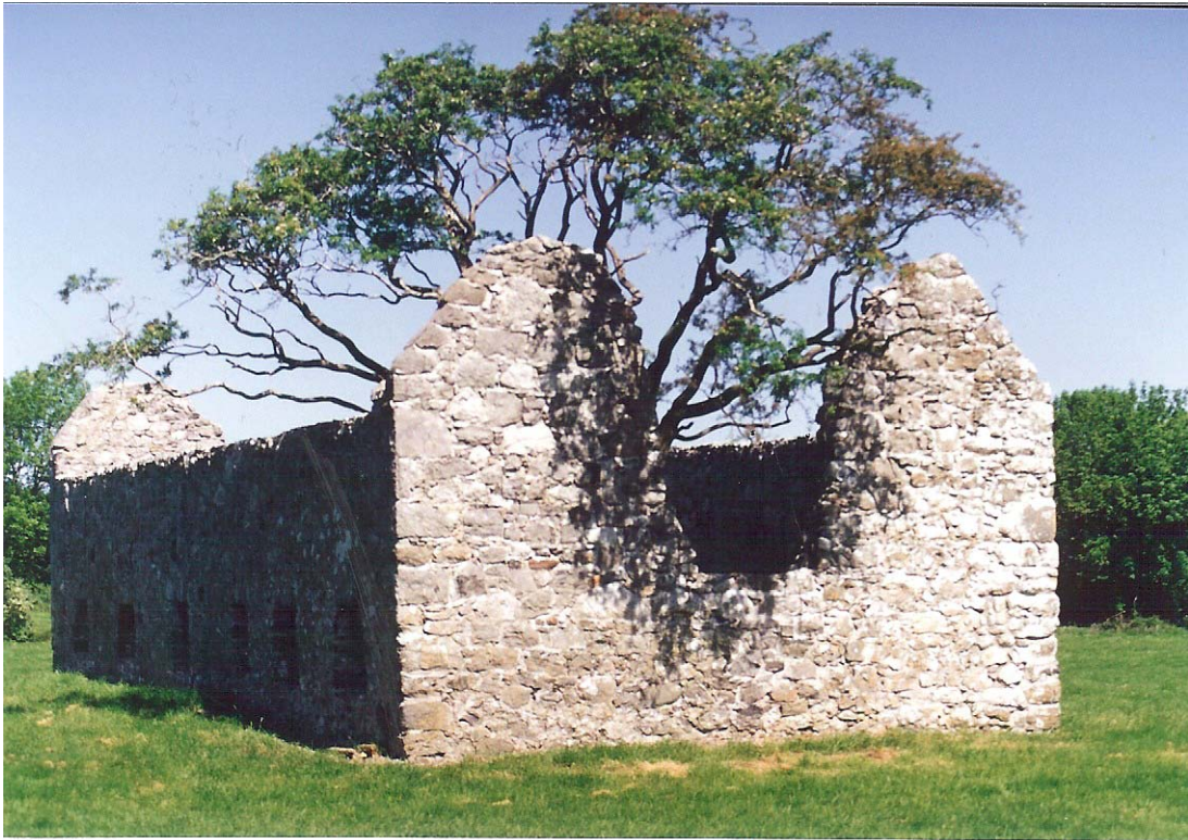
..after restoration work.
